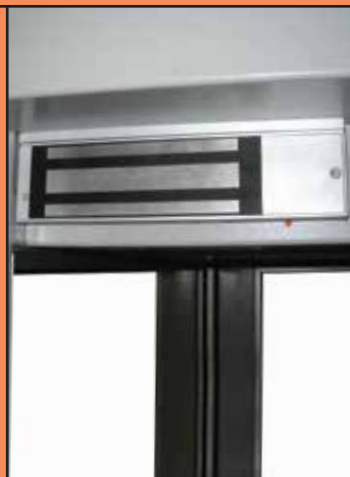
Recessed 500kg monitored magnetic lock
