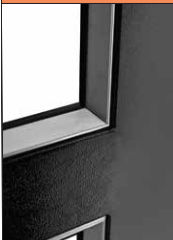
Welded steel frame with aluminium and glass infill
