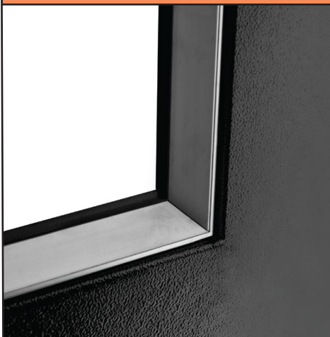
Welded steel frame with aluminium and glass infill
